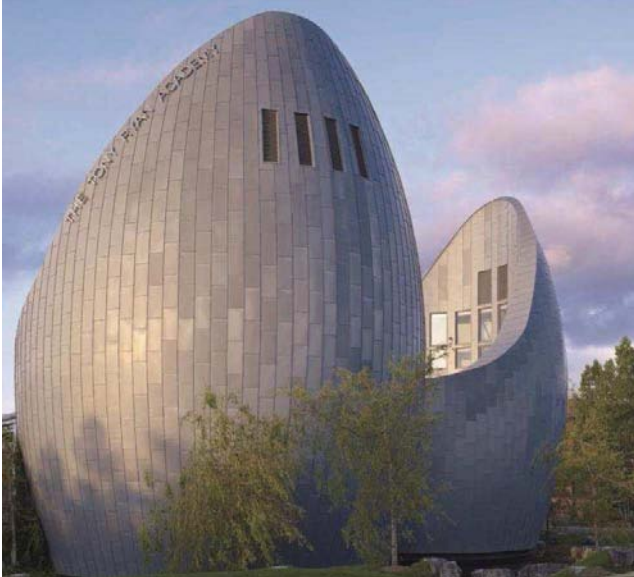
Figure 27. Color difference on stainless steel building exterior of Tony Ryan College in Dublin, Ireland.
