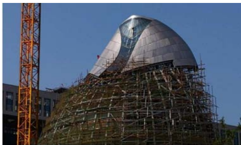
Figure 3. Stainless steel color difference (illuminated face).
