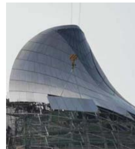
Figure 4. Stainless steel color difference (shady face).
