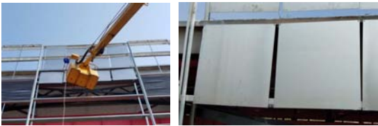
Figure 13. Effect of fluorocarbon spraying on outer surface of stainless steel in high-altitude simulation.
